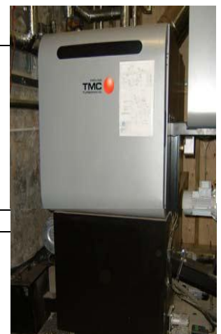
Froling Turbomatic Chip Boiler
